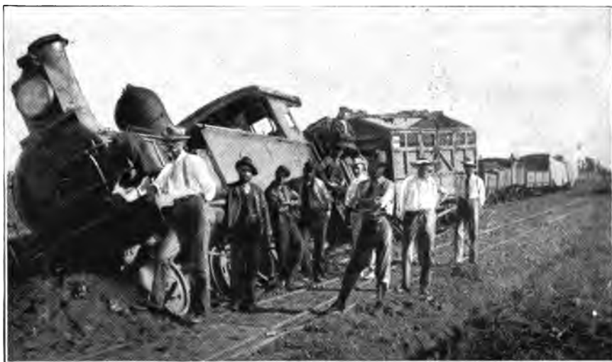
Off the Rails: A frequent Sight on the new Railway.
